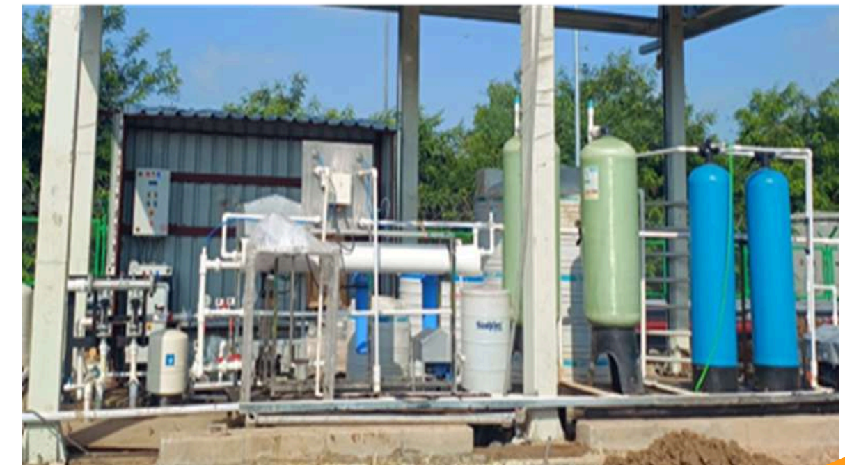
ZLD – Zero Liquid Discharge Plant
