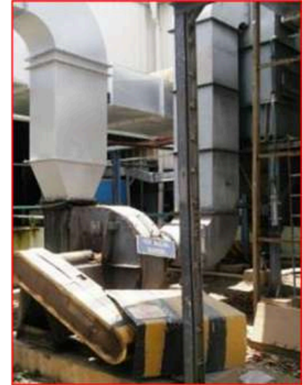
❖ Flow Rate - 12000CMH, Motor - 25Hp & 1455RPM, Blower fan - 1500RPM
