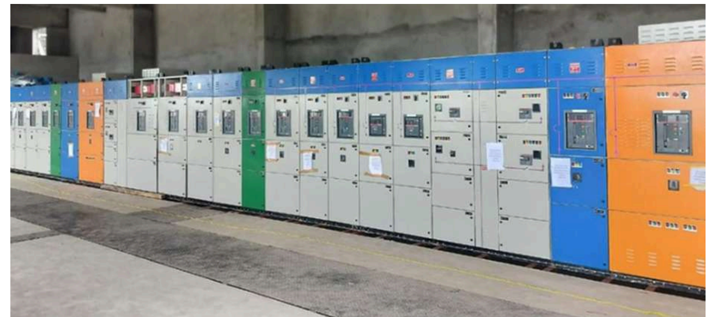
LT PANEL INSTALLATION WORK
