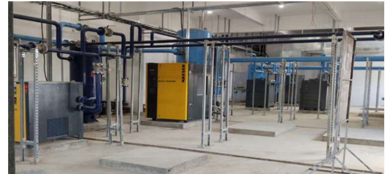
Compressor Installation Work
