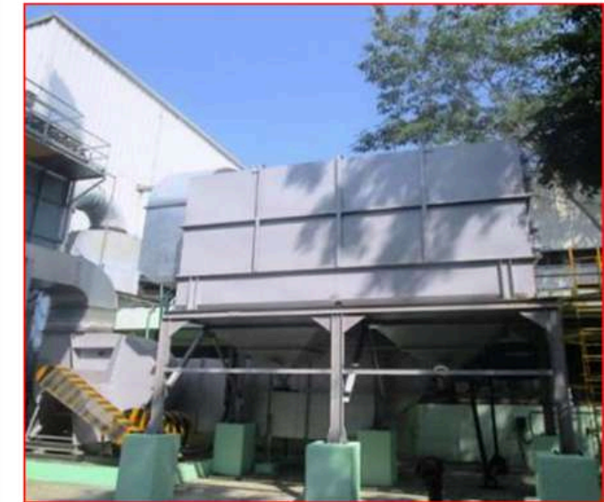
❖ Flow Rate - 40000CMH, Motor - 75Hp & 1460RPM, Blower fan - 916RPM
